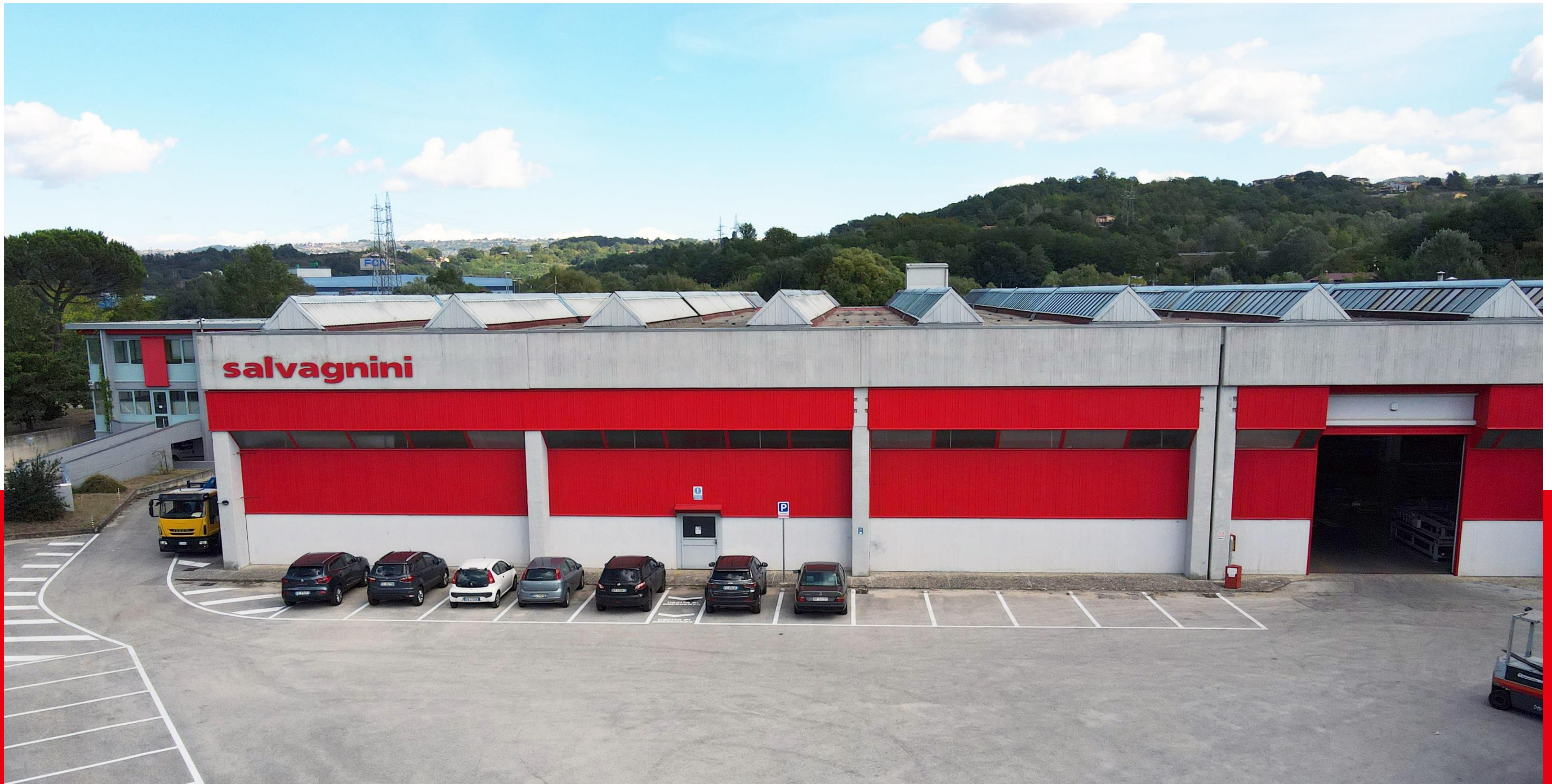
Salvagnini Industriale Handling devices manufacturing
